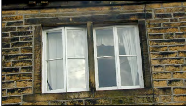
Simple painted timber casement windows, although not original well proportioned and characteristic of the conservation area
